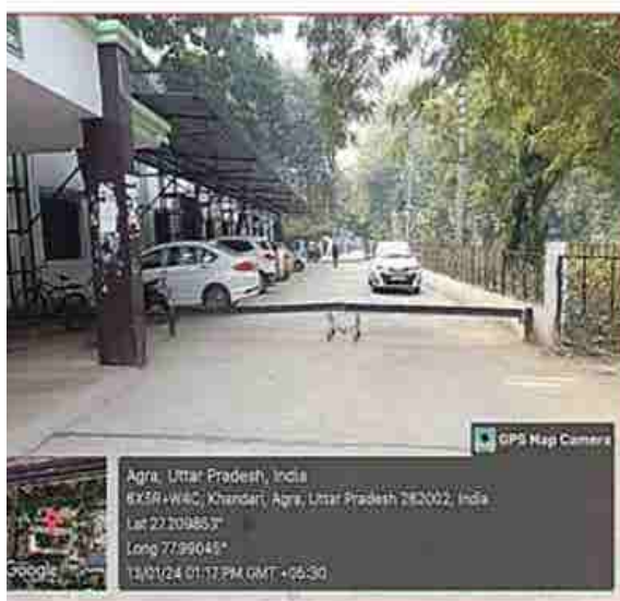
Restricted entry of vehicles
