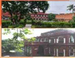
University Administrative Building
