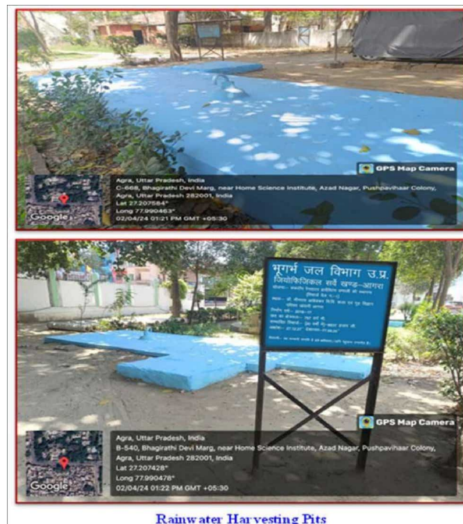
Rainwater Harvesting Pits
