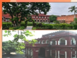
University Administrative Building
