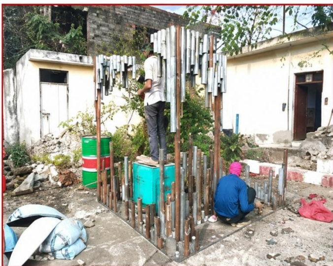
Work in progress on Molding for Cube
