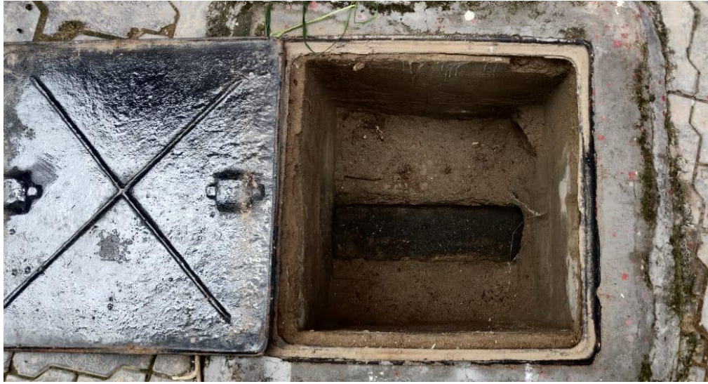
Pic- Groundwater recharge system in IET, Khandari Campus
