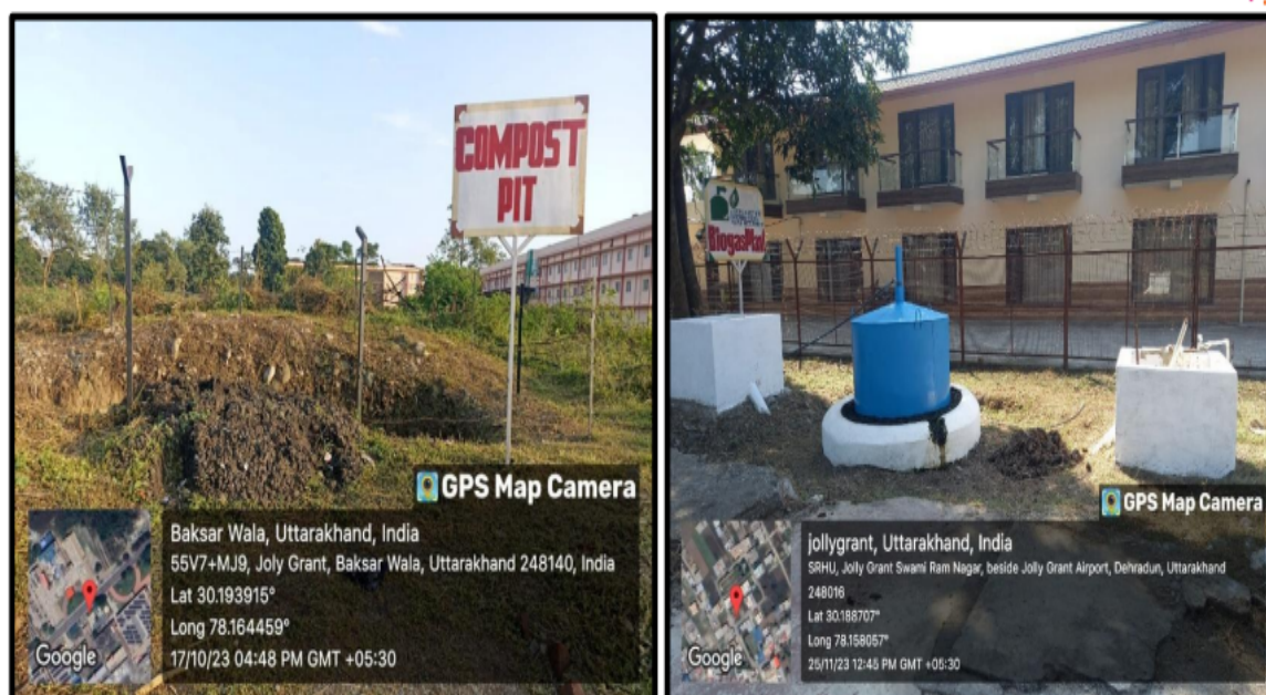
Compost pit and Biogas Plant are located within the university premises
