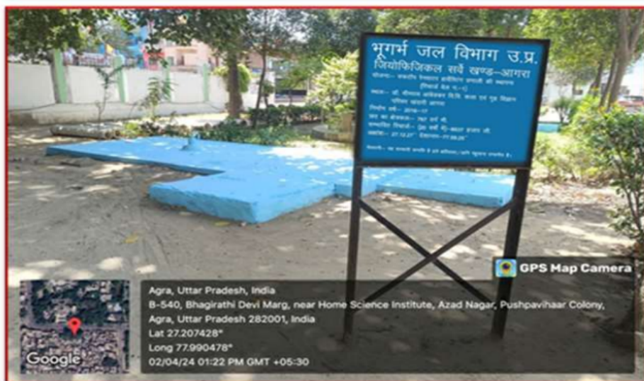
Rainwater Harvesting Pits
